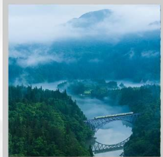
“TADAMI FIRST BRIDGE”
